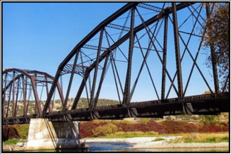
Ririe Pegram Truss Railroad Bridge
