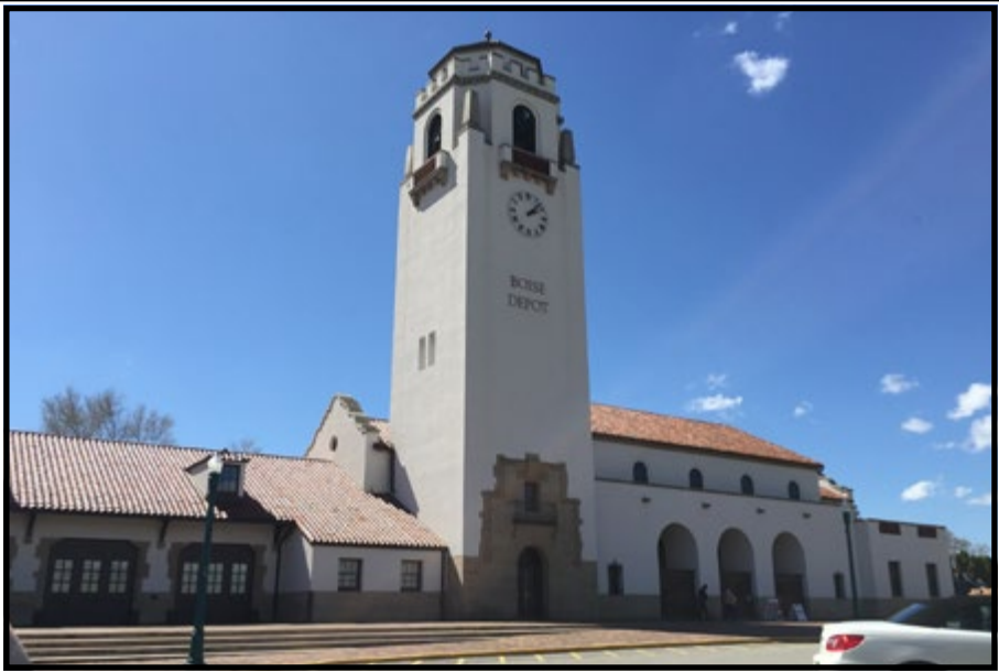
Union Pacific Mainline Depot
