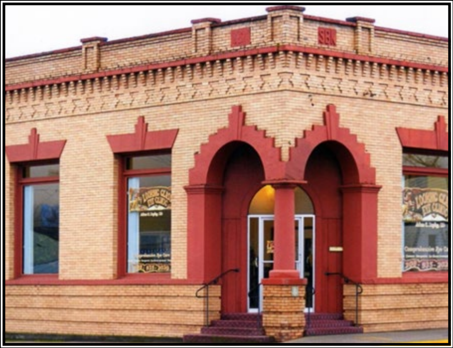
State Bank of Kamiah
